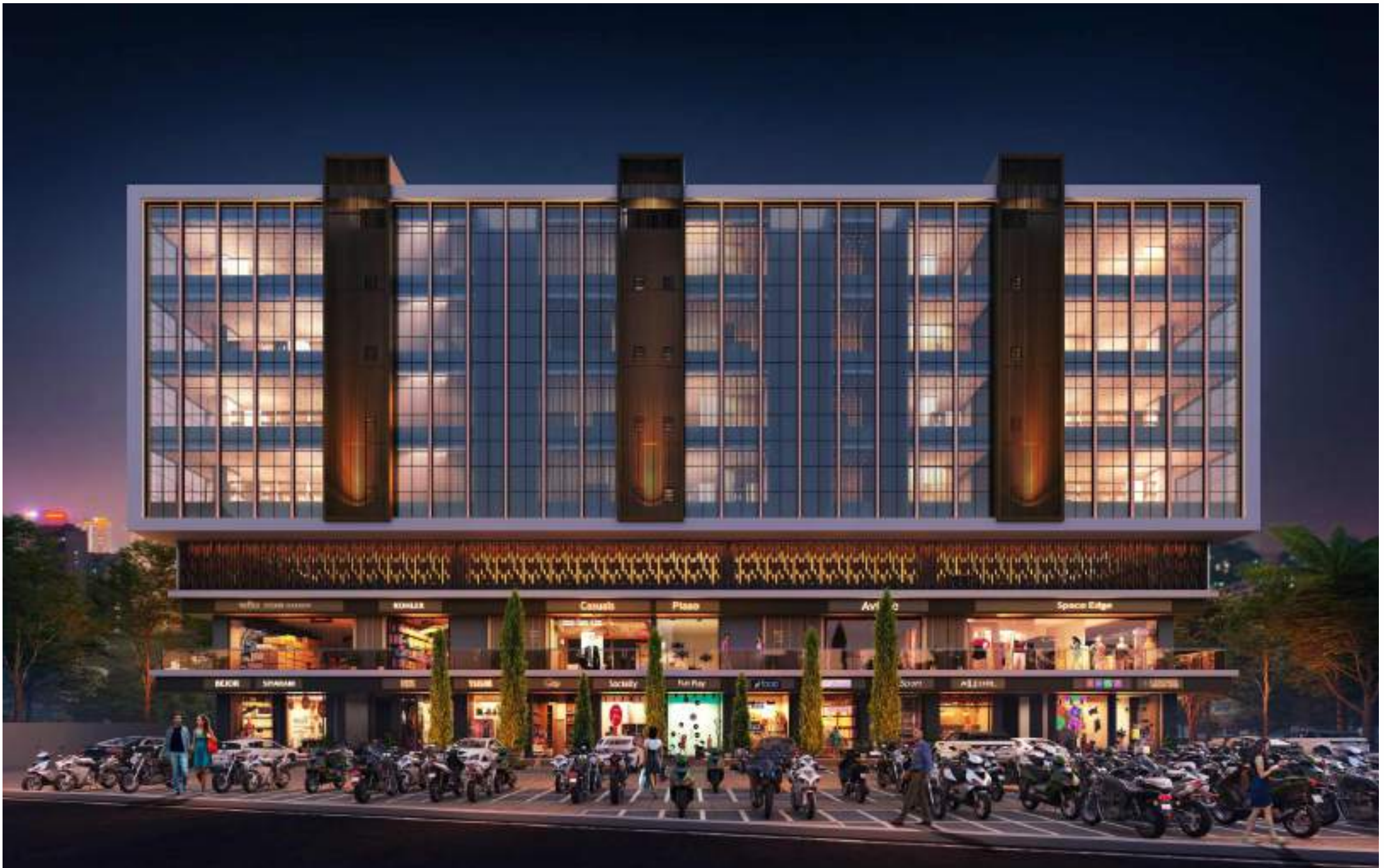
PrestigeChambers PHASE - II
